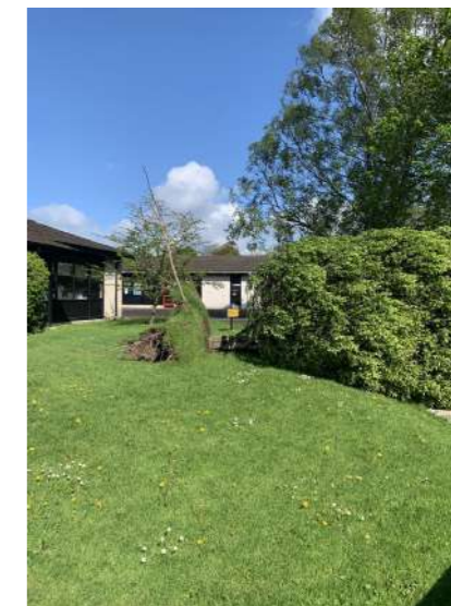
Damage caused by Storm Hannah
